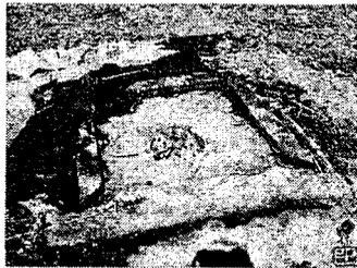
Figure 4. Redwood strips surrounding the inlet/outlet structure at bottom of pond
