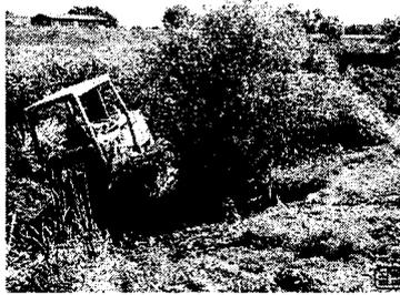
Figure 2. Willow tree and cattails being removed to exhume the PVC Geomembrane
