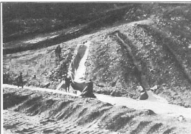
Photo 1. Downstream drain during geotextile filter placement.
