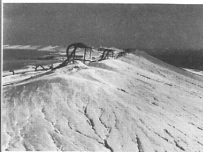
Photo 1. ERGO Tailings dam - Tailings deposition through hydrocyclones.
