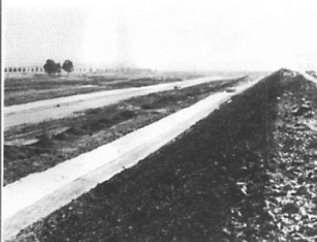
Photo 2. Filter drains under construction outside earthfill starter wall.
