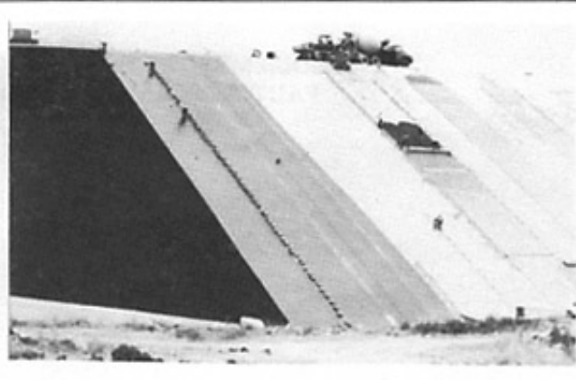
Photo 2. Codole dam: placing of upstream geomembrane.
