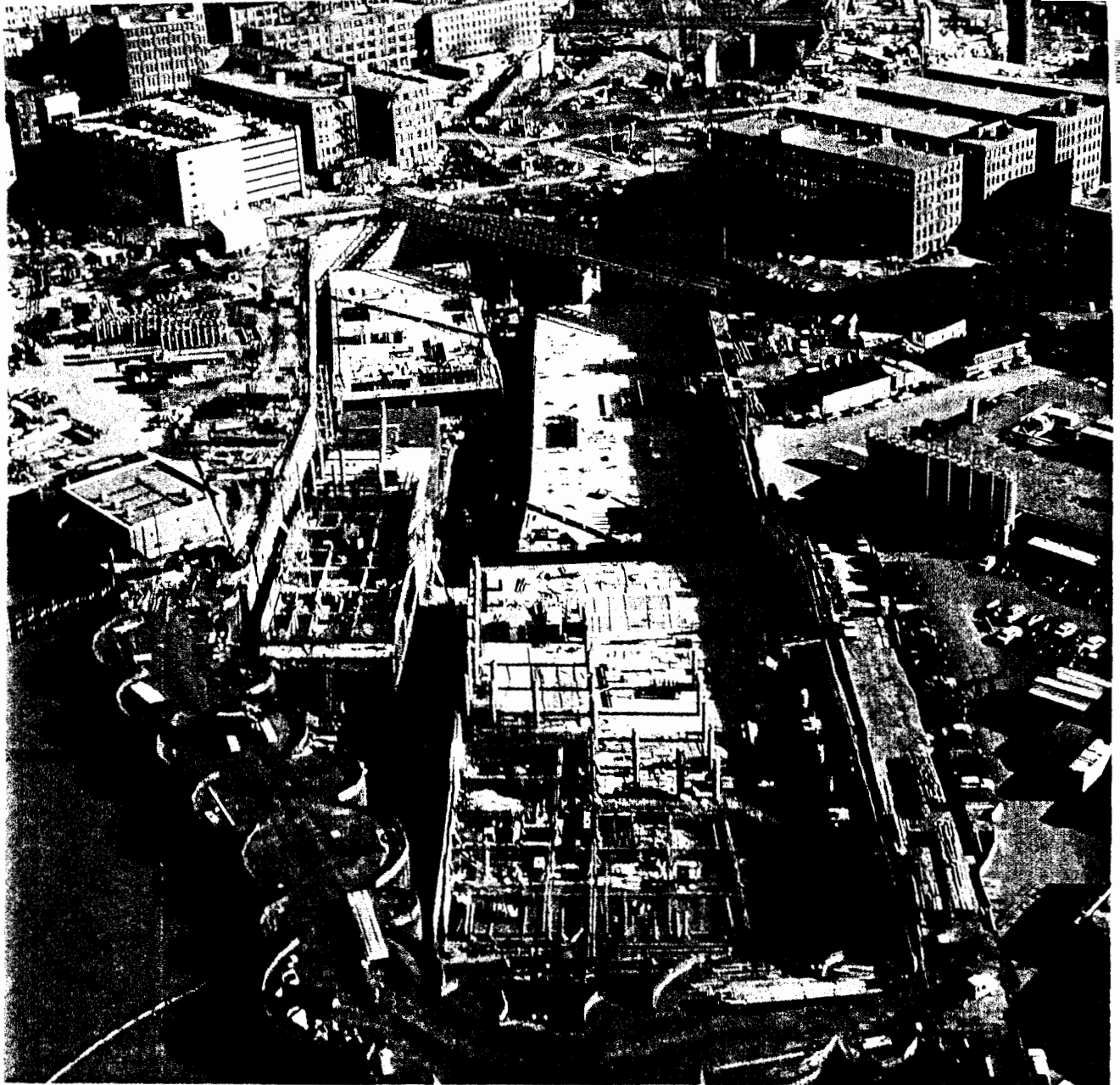
Photo 1. A giant cofferdam in Fort Point Channel creates a casting basin for the approximately 450-ft long immersed tunnel tubes
