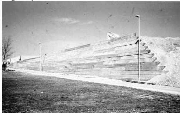
Figure 14: “Unterkaka”: reinforced slope and platform nearly completed
