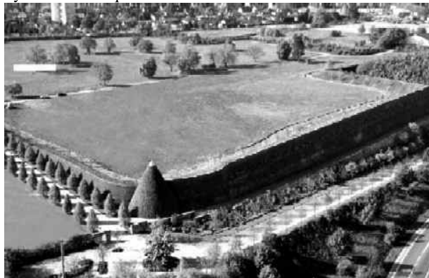
Figure 16: "Lobbe Holding": completed platform and reinforced slopes
