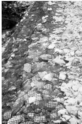
Figure 12: “Federal Road B 277”: extremely coarse fill confined by flexible geogrids
