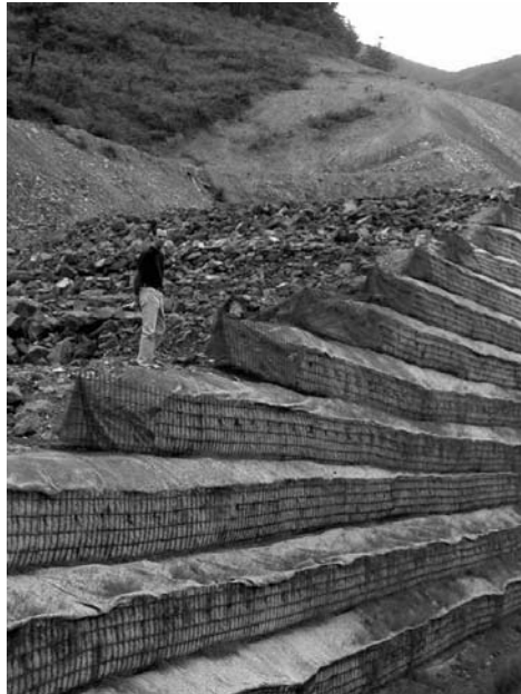
Figure 18: “Etxegarate”: construction stage; note the big vertical spacings
