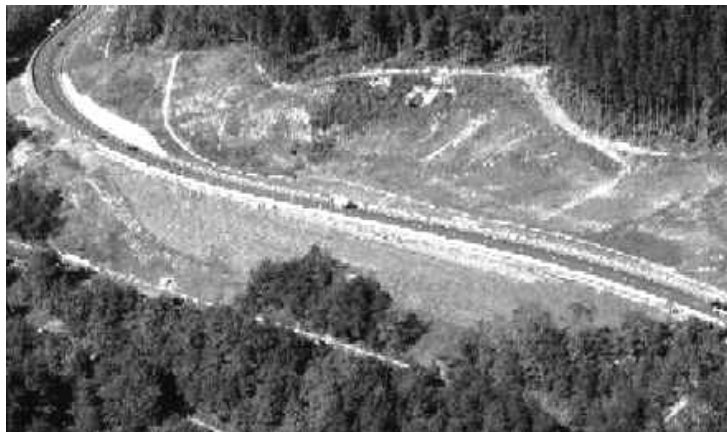
Figure 19: “Etxegarate”: structure just after completion
