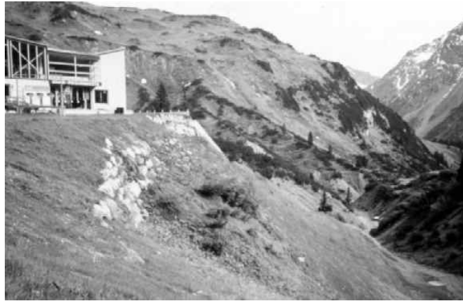
Figure 10: “Steinmaderer Wand”: one year later – the structure has become a part of natural landscape
