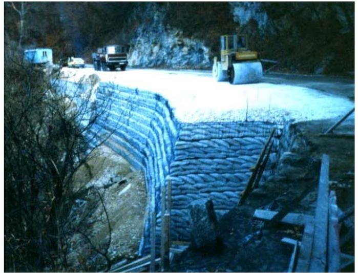
Figure 8. Jugovsko Hanche: completing landslide stabilization and road widening (before installation of the final Muralex® facing)
