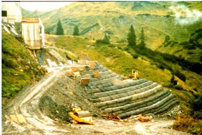
Figure 3. Steinmaderer Wand: construction stage of stabilizing reinforced slope (1994)
