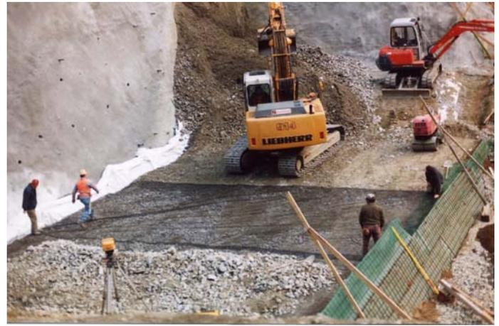
Figure 11. Gondo: start of construction; Fortrac®200-geogrid, fill layers and facing installation
