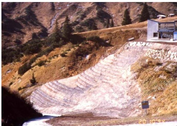
Figure 4. Steinmaderer Wand: slope reconstruction just after completion (1994)
