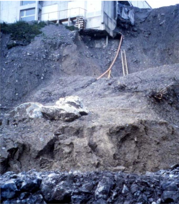
Figure 1. Steinmaderer Wand, Austria: Lift-station endangered after failure of landslide mass (1994)
