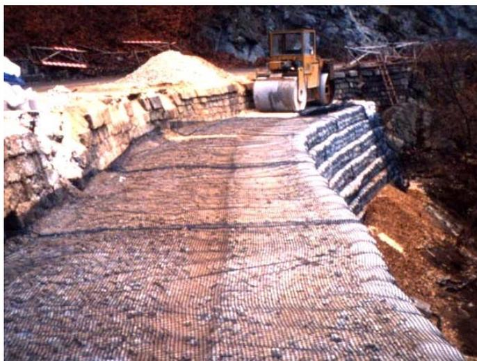
Figure 7. Jugovsko Hanche: construction of geogrid-reinforced wall, top part of old stone masonry retaining wall to the left
