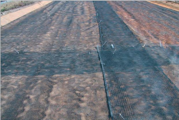
less than 7.5 cm, due in large part to the reinforcement enhancement provided by the **Fornit® 30** geogrid. The contractor was able to begin compaction to final level within two weeks and completed work on the base phase more than a month ahead of schedule.
