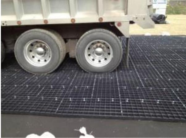
Figure 6 A well pad system that consists of a 1.5mm (60-mil) HDPE textured geomembrane, a 340 g/m<sup>2</sup> (10 oz/yd<sup>2</sup>) cushion geotextile, a 50mm (2in.) recycled foam product and a durable, reusable specialty mat product. Andrejack-Loux and Filshill, 2013
